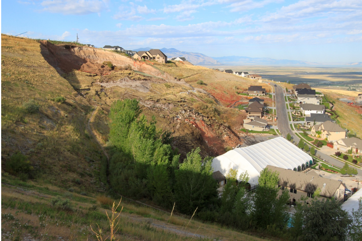
Figure 2-1: North Salt Lake Landslide (Beukelman, 2014)
